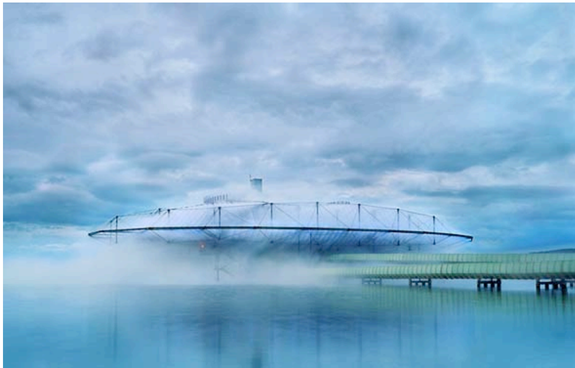
Fig. 7 Diller & Scofidio Blur Building Expo.02 Yverdon-les-Bains
